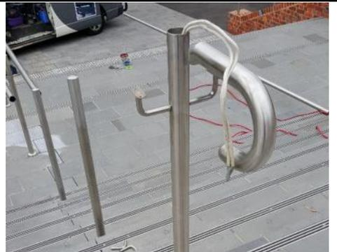
We custom made special pins, including a select number of hollow pins. We then cut out 3 meter sections of the existing rail and welded in our patented slotted rail. This made fitting our lighting a breeze, and the results speak for themselves.
