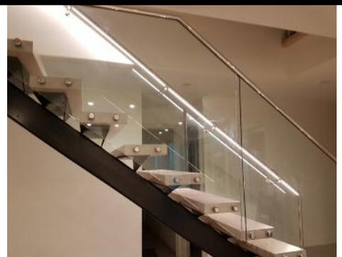
In the case of the Classic Slimline, we are not able to use our patented hollow brackets for wiring. In this particular application we were able to feed our wiring up through a post at the bottom of the stairs, which then continued as the handrail.
